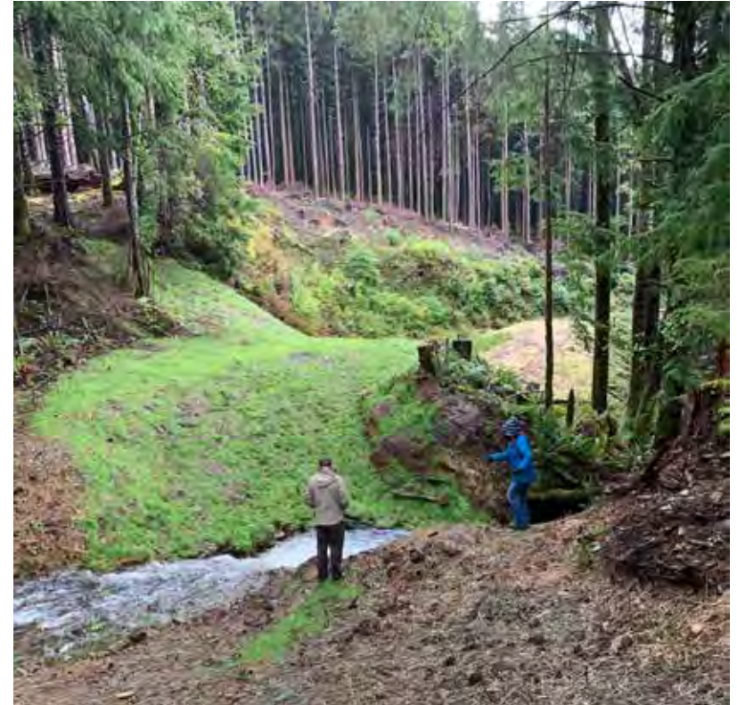
Example of where a culvert located under a logging road was removed. Without vegetation to stabilize the soil along the creek, erosion can increase.
